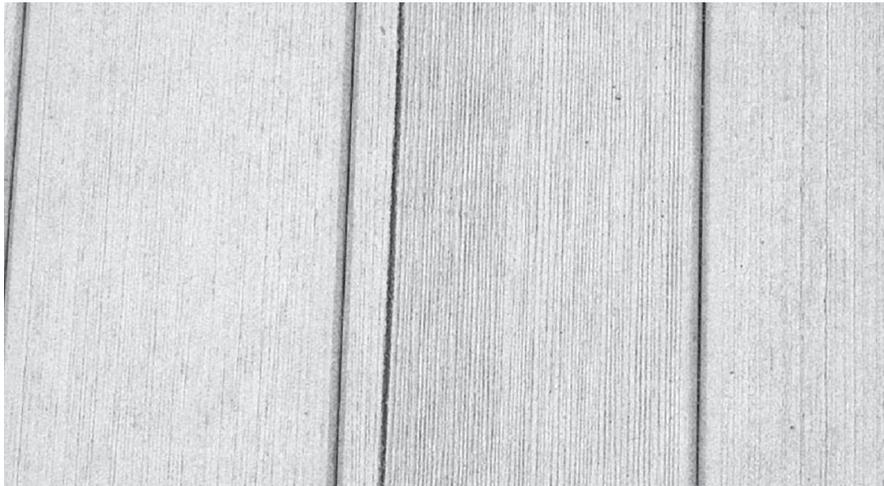
**Figure 12.6** A crack in a composite deck board as a result of buckling due to water absorption and insufficient gapping.
