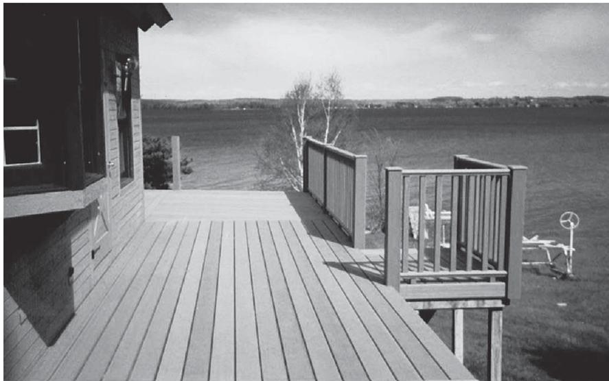
**Figure 12.1** A typical gapping of deck boards on a deck.
