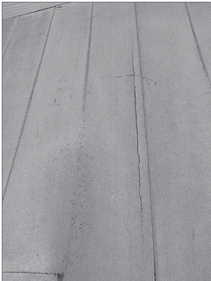
**Figure 12.5** Moisture-induced distortion and mechanical failure of WPC deck boards.
