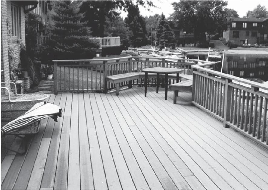
**Figure 12.2** A typical gapping of deck boards on a deck.
