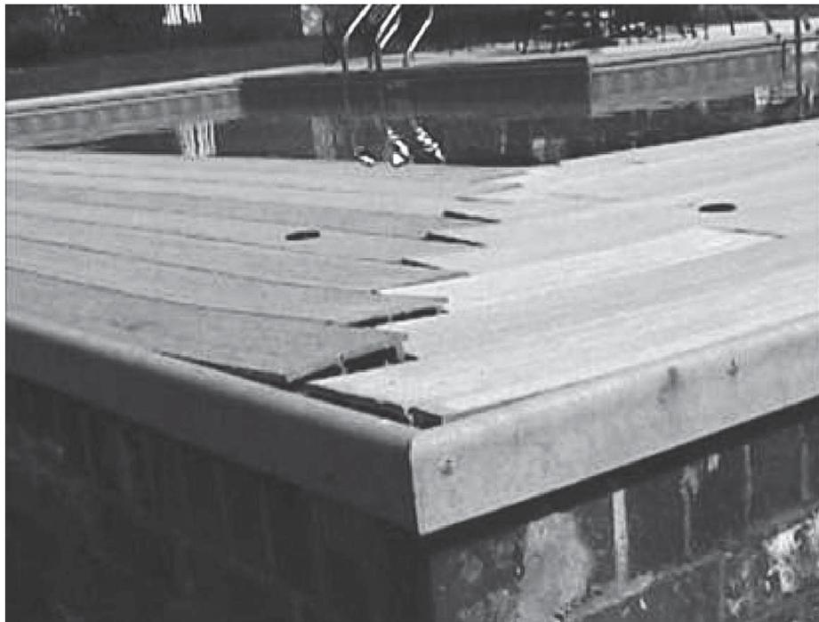
**Figure 12.7** Moisture-induced dimensional instability of a WPC material.
